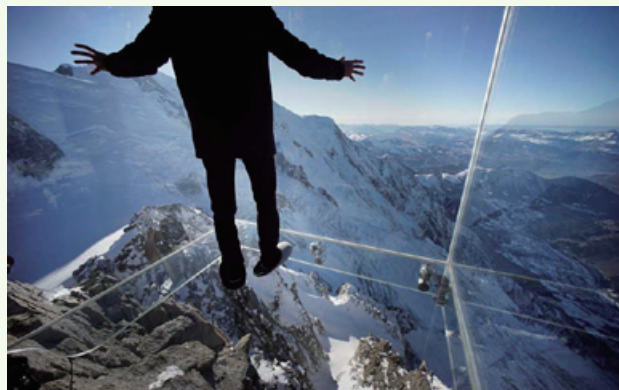
Project "The step on the Void" - France l'Aiguille du Midi. Pilkington Optiwhite™ 12mm, toughened, heat soak tested and laminated by a French glazier with interlayer Sentry Glass type. Photo © Joelle Bozon.
